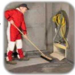
Sweep Chute Wall Panel
